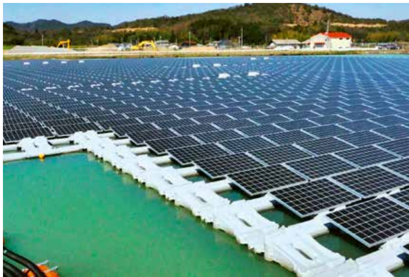
Floating solar Photovoltaic panels to meet peak demand
